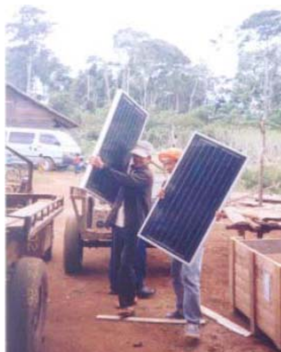
Small PV power installation in Vietnam
