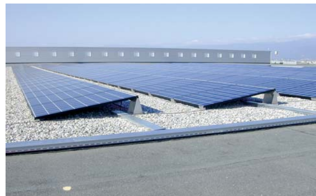
70 kW p roof system at Geneva exhibition centre
